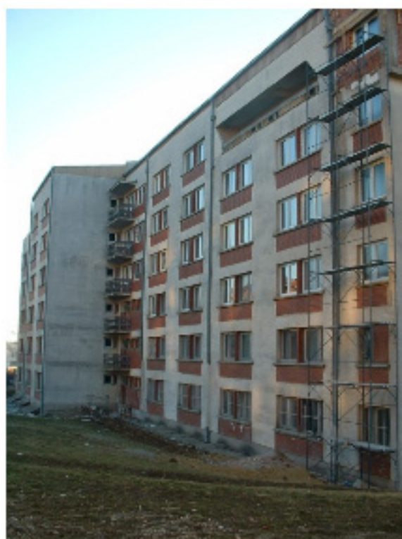
Dormitory Prishtin -Block 5
