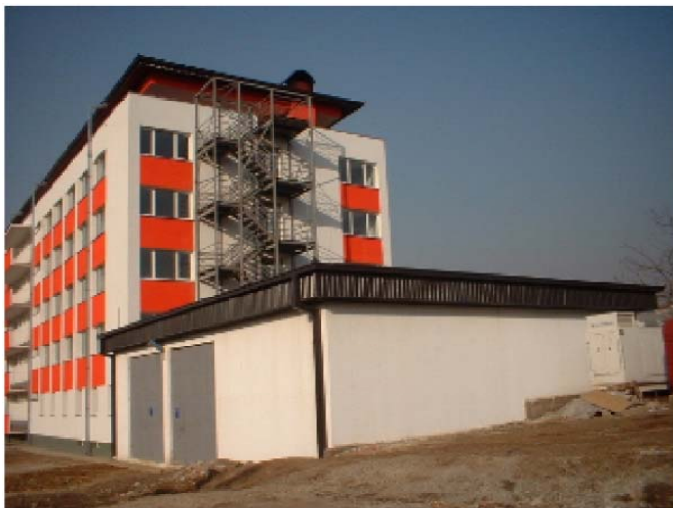
Dormitory Prishtina - Bojler Room at Block 1
