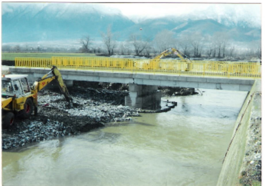
Ura - Bridge in Peja L=2 \times 12 \text{ m}' = 24 \text{ m}'
